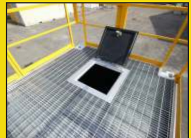
Roof Access Hatch
