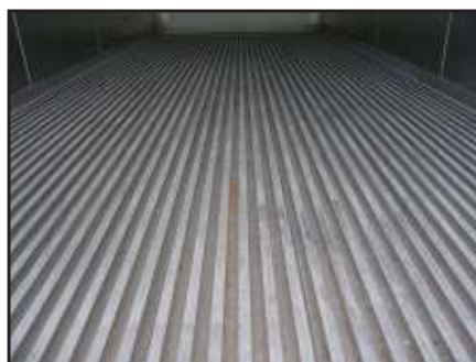
T-shaped decking distributes chilled air from the floor
